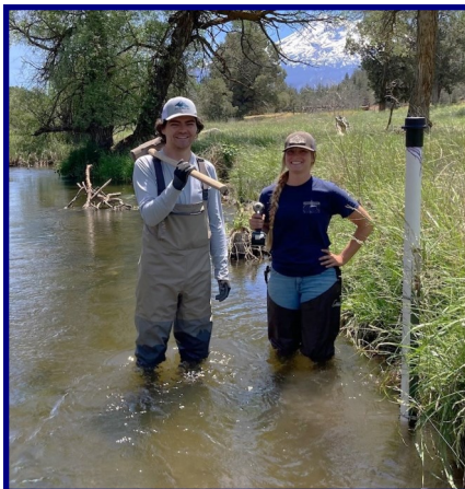
Jose and Mallory installing a stilling well to track flows and measure project efficacy in the Upper Shasta River.
