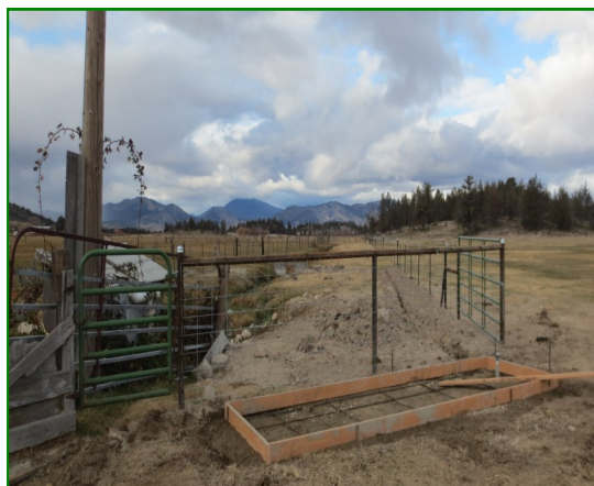
Above: Stockwater under construction
