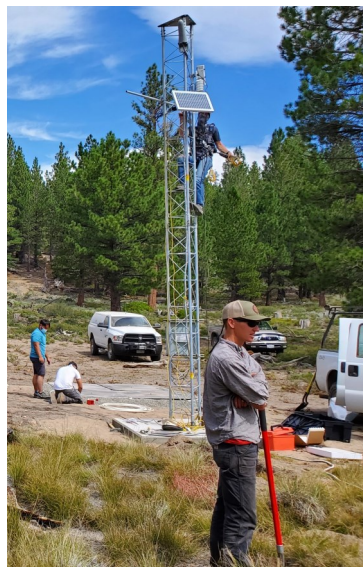
HyDAS Station Construction at Bolam
