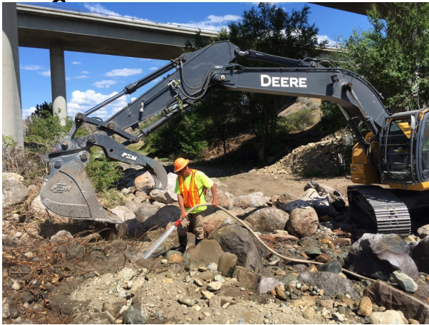
North Rivers Construction placing boulders with Hwy 15 in the background
